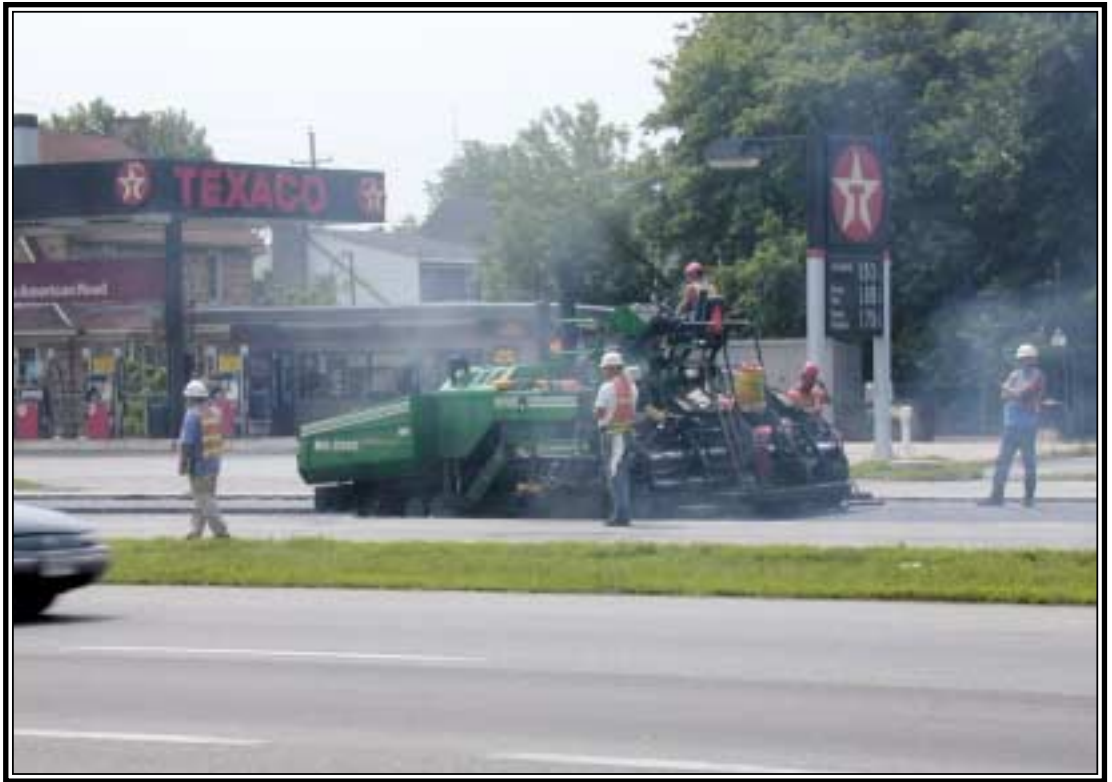
Superpave replaces deteriorated concrete at Landing Road.
