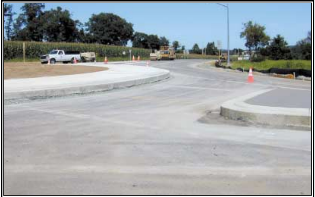
Raised concrete islands direct traffic, accommodate signing and are used as landscape planters.
