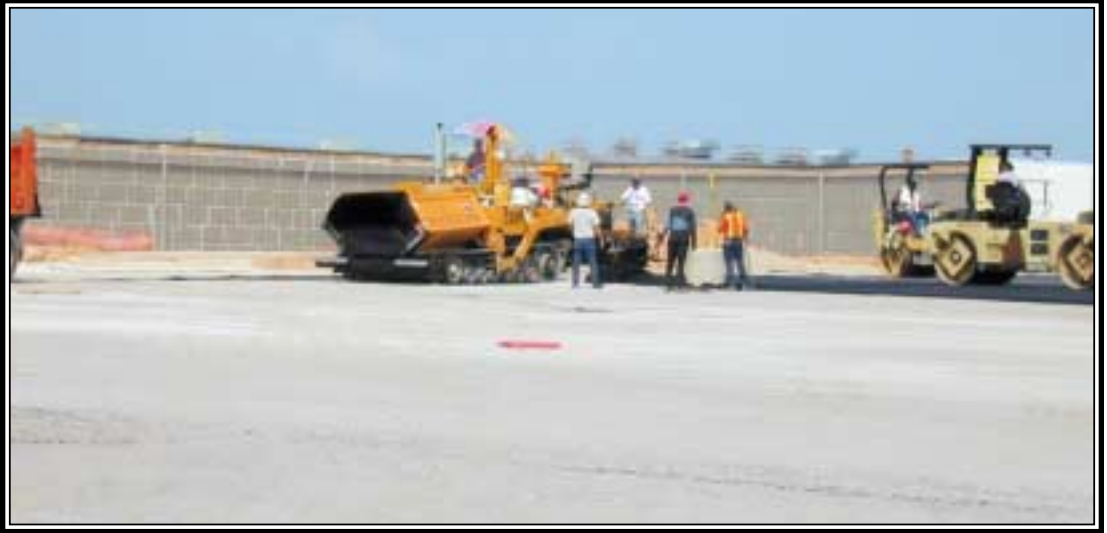
Track Paver places initial base course of HMA.
