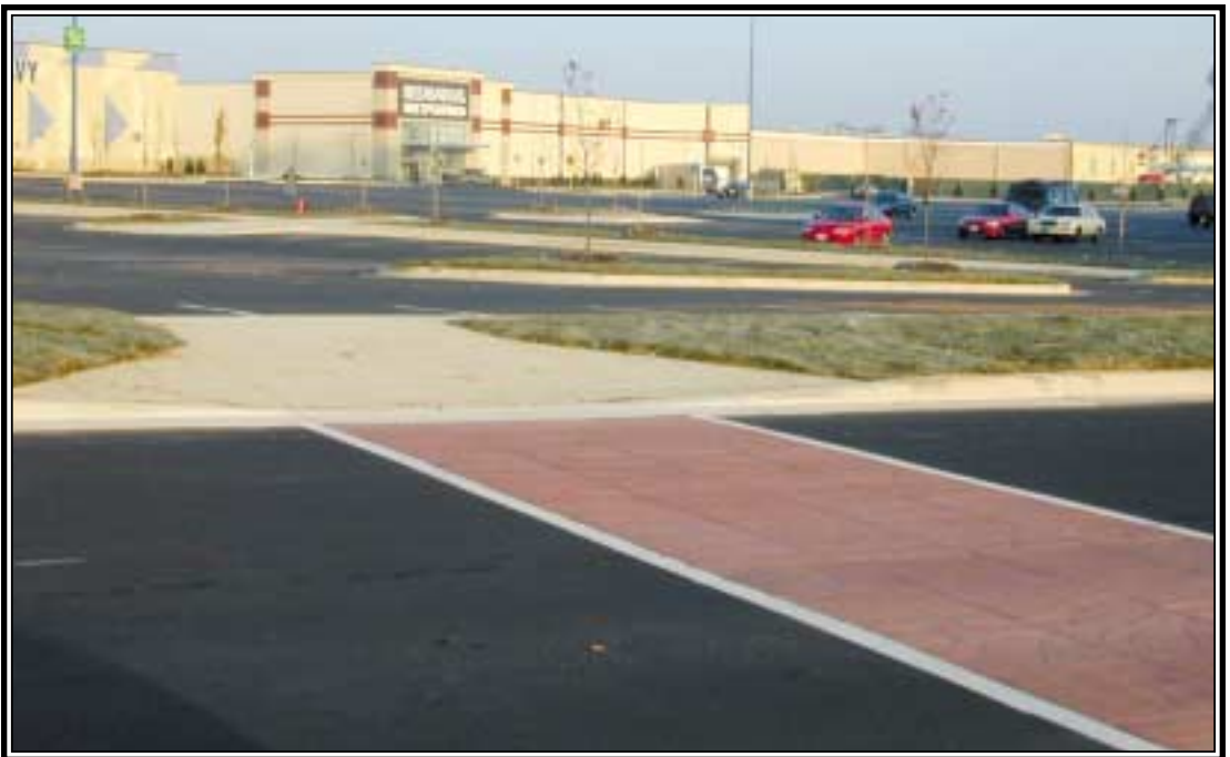
Cross walks are clearly delineated by colored pavement.
