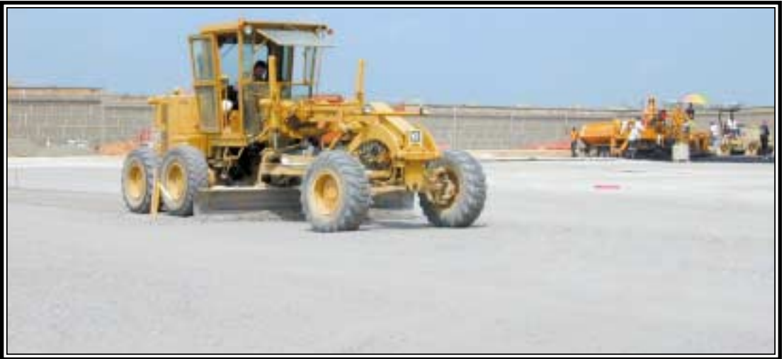
Conventional fine grading techniques were utilized to insure positive drainage.
