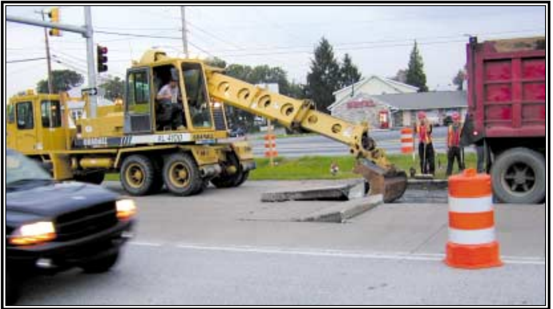
T.C. Simons crews remove 6 1/2" whitetopping at US 40 & Landing Road.
