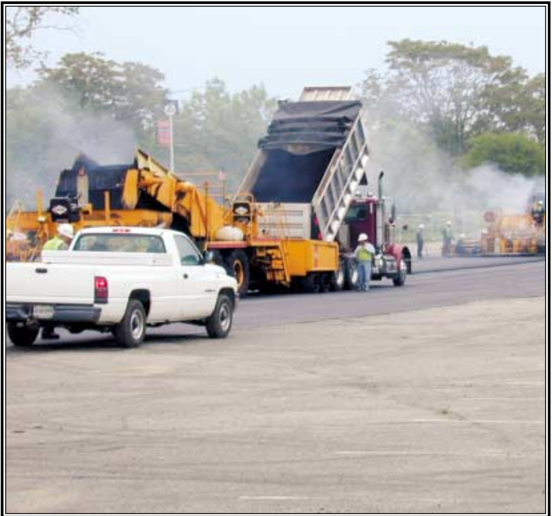
Staggered paver operation allowed construction of a hot longitudinal joint.
