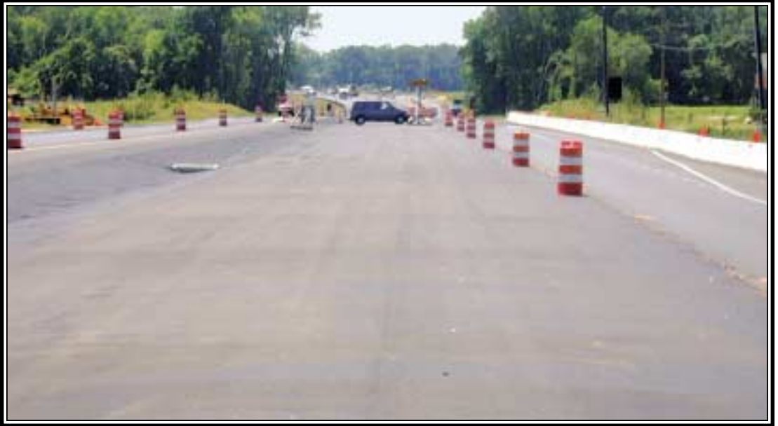
Newly paved roadway prior to traffic switch uses 12.5 Superpave surface.
