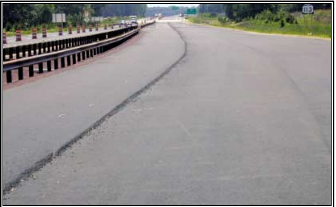
Extensive cores were taken in order to verify longitudinal joint densities.
