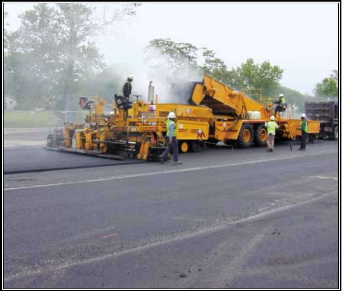
Echelon paving train includes two Blaw-Knox material transfer devices.
