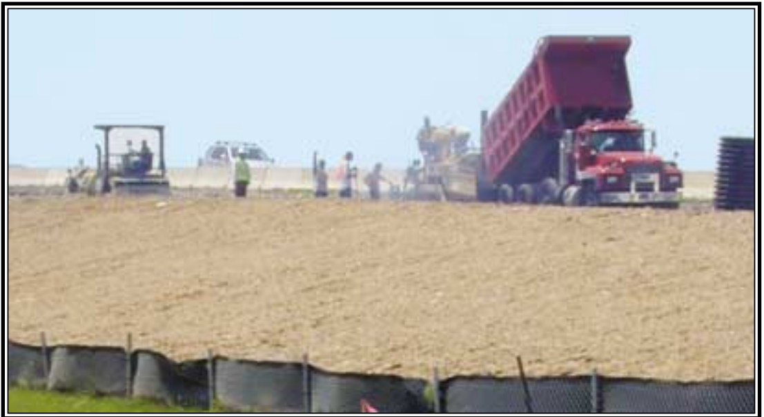
Complete paving train works to relocate roadway over newly constructed fill.
