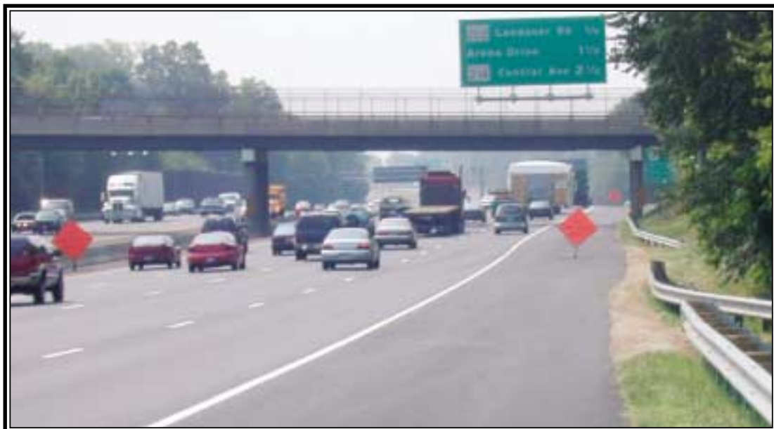
The Capital Beltway carries 187,000 VPD at this location making maintenance of traffic extremely difficult
