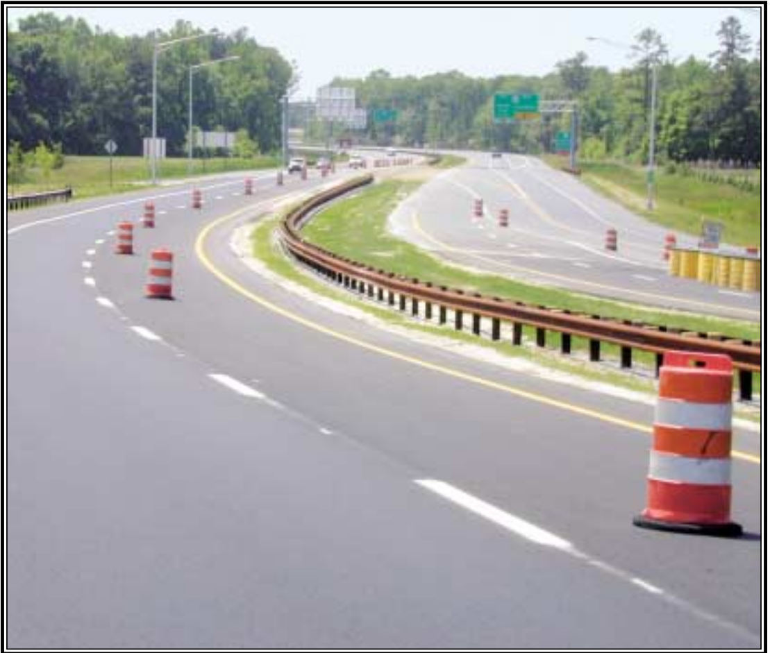
Divided roadway section uses paved drainage flumes and weathered steel median barriers.
