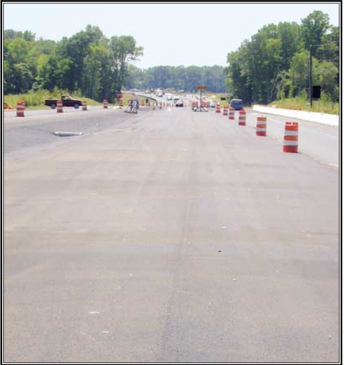
New surface pavement prior to opening to traffic.
