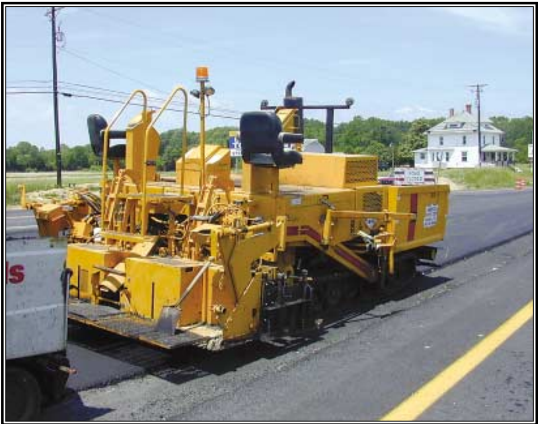
Blaw-Knox paver was used to place Superpave mixture.
