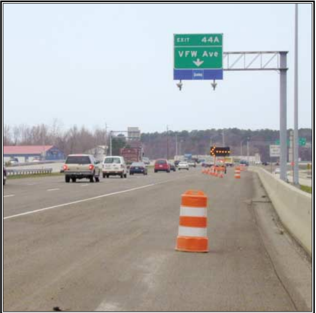
Finish ground roadway prior to paving.
