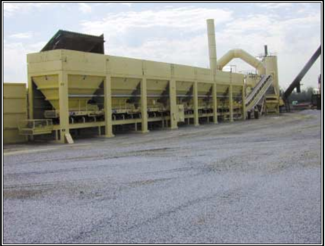
New plant utilizes seven cold feeds and a rap feeder.
