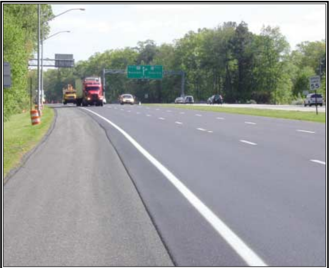
9.5 mm Superpave intermediate course prior to SMA placement.
