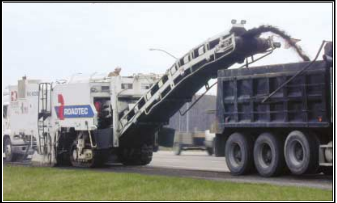
Carbide grinding operation by Dixie Construction Co., Inc..
