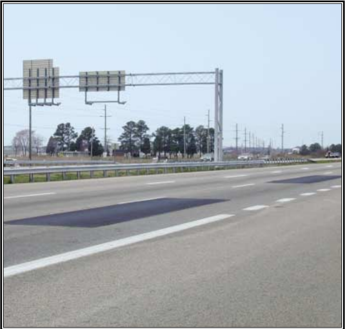
Partial depth patching WBL US Route 50.
